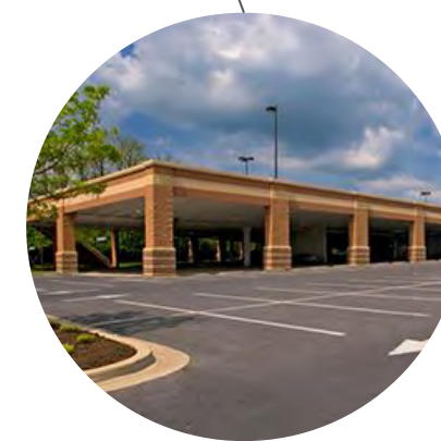
SECOND STORY PARKING STRUCTURE
