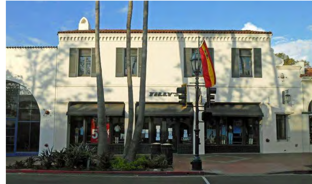
EXISTING STATE STREET FACADE
