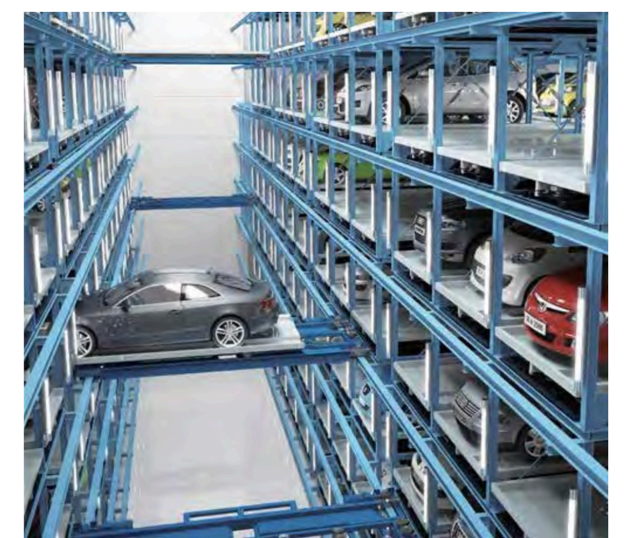
AUTOMATED PARKING CAN REDUCE SPACE PER CAR BY UP TO 50% WITH 2-3 MINUTE RETRIEVAL TIME
