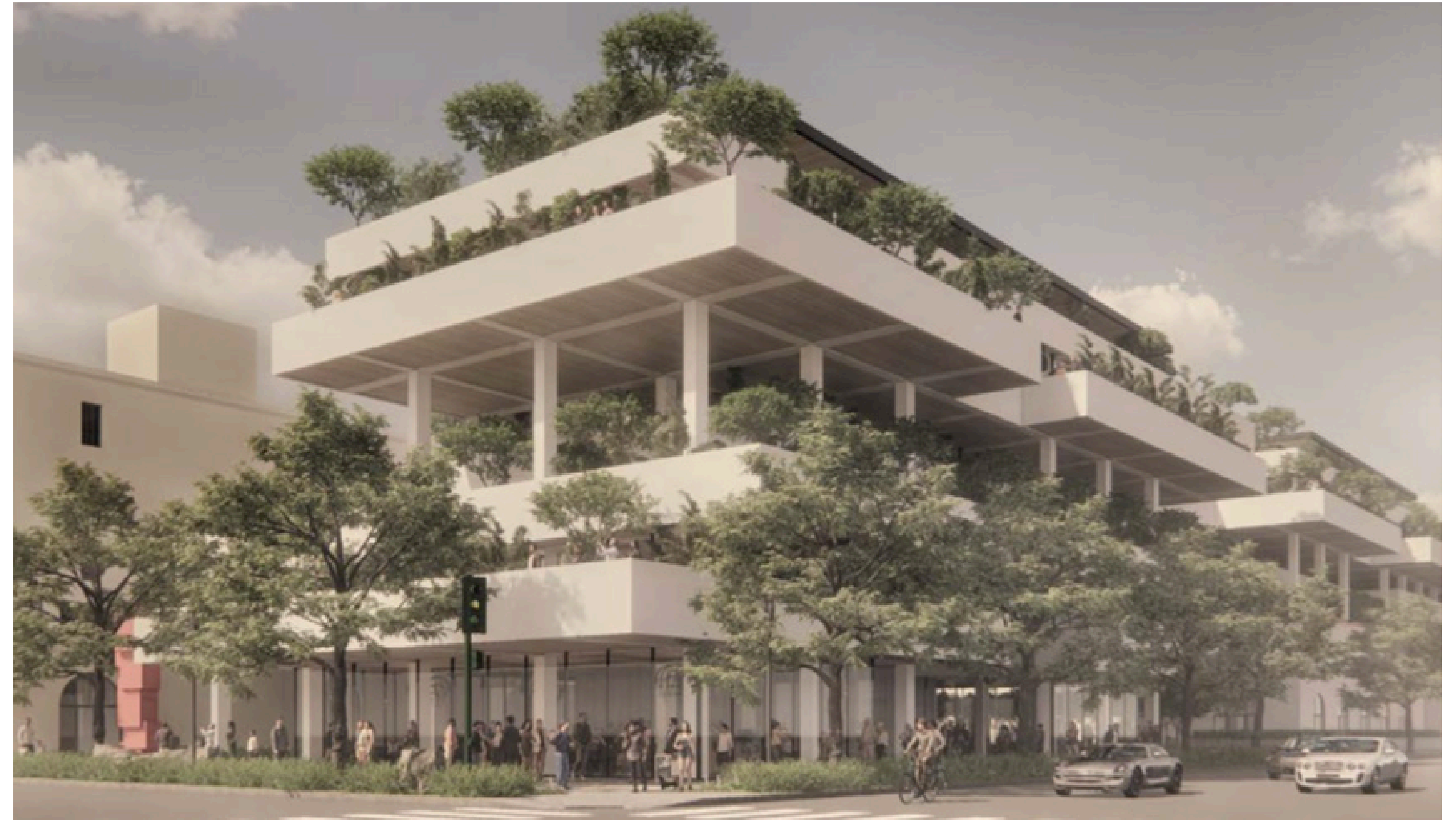
STORM WATER RETENTION IN 1" RAIN EVENT, 21,817 GALLONS ON UPPER LEVELS AND 4,675 ON GROUND LEVEL
