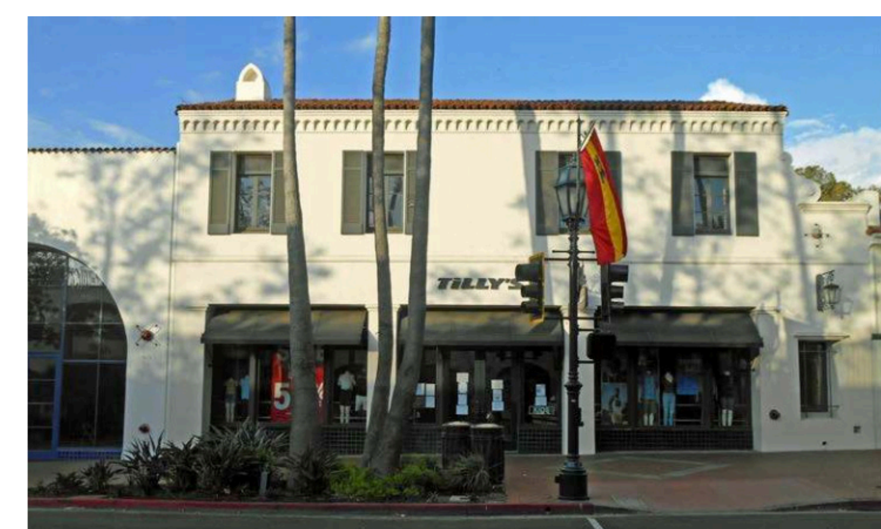
EXISTING STATE STREET FACADE
